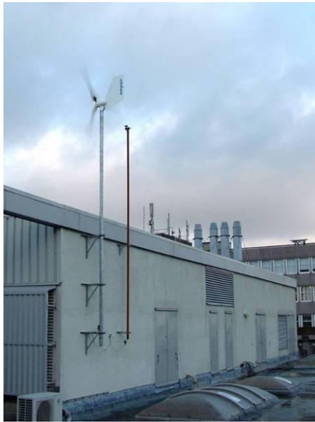
This turbine is being monitored by Napier University. The hub height is approximately 2m above a flat roof. The building is around 25m tall but it is surrounded by other tall buildings.
