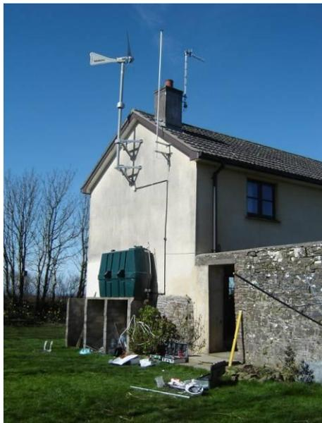
West Staddon Farm is a farm house located in north Devon close to the coast. This is the latest Windsave mounting system with a mass damper attached to the pole to reduce vibrations.
