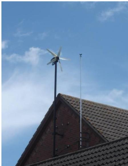
This turbine is installed on a modern detached house and is mounted on the gable end. There is a large open field to the south west of the property. To the north of the house is an urban area.
