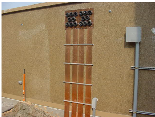
16 Port PEEP on Equipment Shelter
