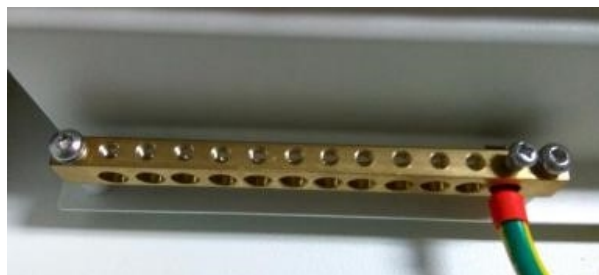
Figure 3.9 Grounding terminal block on the metal bracket
