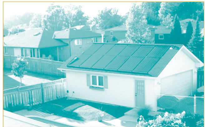
Welland, Ontario. This 5-m x 10-m (16-ft. x 32-ft.) free-form pool is heated by six 4.4-m 2 (4-ft. x 12-ft.) solar collectors mounted on the garage. Photo courtesy of Daystar Energy.
