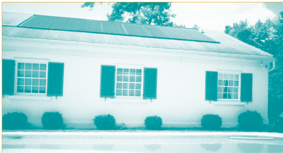
Ottawa, Ontario. 6.1-m x 12.2-m (20-ft. x 40-ft.) in-ground pool, eight 4.4-m 2 (4-ft. x 12-ft.) solar collectors. Photo courtesy of Heliocol Canada.
