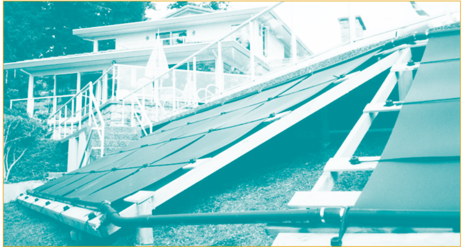
7 White Rock, British Columbia. Eight 4-m 2 (4-ft. x 10-ft.) solar collectors on a wooden ground rack. Photo courtesy of Taylor Munro Energy Systems.
