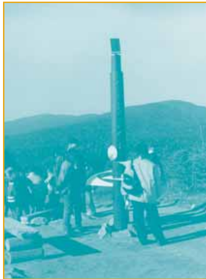
S A small PV module is used to power a trail indicator at night at Mont-Tremblant, Quebec. Photo courtesy of TN conseil inc.
