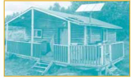
S Remote residences or cottages can have access to electricity without extending the grid. Photo courtesy of Solener Inc.
