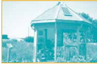
S Water oxygenation compressors and water pumps are examples of PV systems that function without batteries. Photo courtesy of
