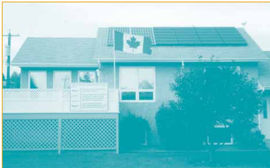
S This house in Edmonton, Alberta, is equipped with a 2.3-kW system that is connected to the local power utility. About 2500 kWh are produced each year. The investment cost in 1995 was $28,000.
