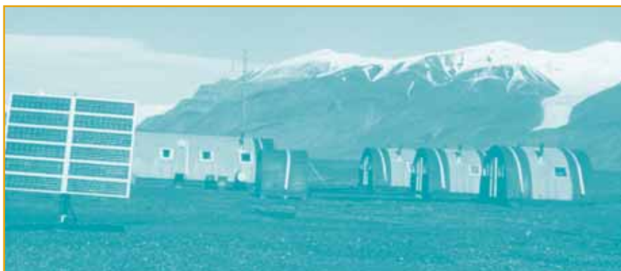
5 Parks Canada's remote camp located in the far north on Ellesmere Island, Nunavut, is powered by a PV array (on a tracker) combined with a wind generator and a gasoline generator.
