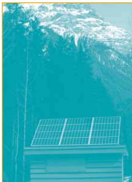
S The autonomous PV system in Yoho National Park, British Columbia, supplies electricity for the amphitheatre projector and recharges the batteries of a golf cart that the staff uses to collect camping fees. Photo courtesy of Sovran Energy Inc.
