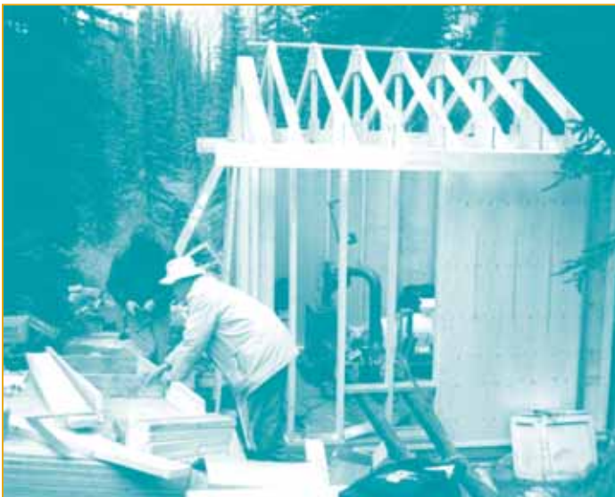
Figure 28. Powerhouse under construction for a 12-kW system (photo courtesy of Thomson and Howe Energy Systems Inc.)
