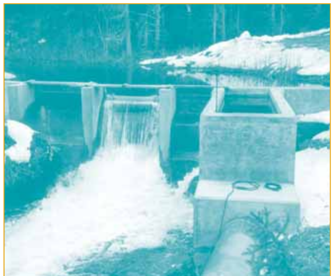
Figure 31. Headwork structure and screen in Morehead Creek, British Columbia (photo courtesy of Thomson and Howe Energy Systems Inc.)
