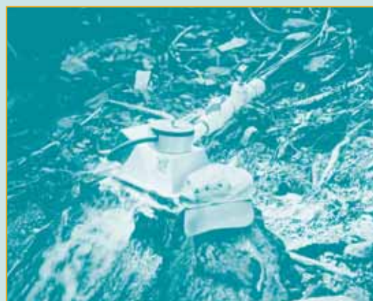
Figure 25. A 200-W micro-hydropower system in action (photo courtesy of Scott Davis, Yalakom Appropriate Technology, British Columbia)
