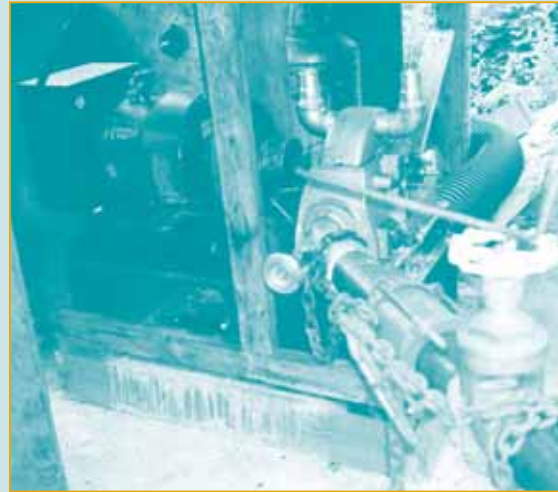
Figure 27. A 10-kW micro-hydropower system in action (photo courtesy of Scott Davis, Yalakom Appropriate Technology, British Columbia)
