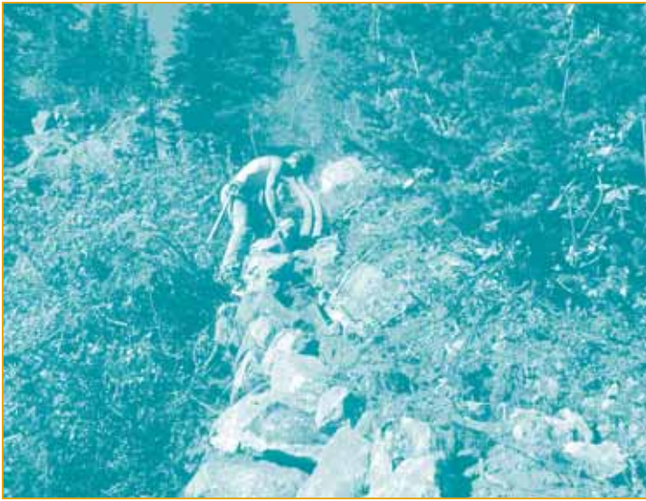
Figure 14. High-density polyethylene (HDPE) penstock being buried in a steep hill (photo courtesy of Thompson and Howe Energy Systems Inc.)
