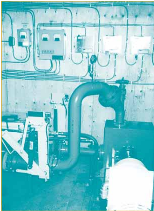
Figure 30. Equipment inside a powerhouse (photo courtesy of Thomson and Howe Energy Systems Inc.)
