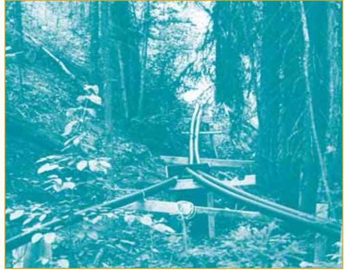
Figure 15. Double 10-cm (4-in.) HDPE penstock pipe for an 8-kW system
