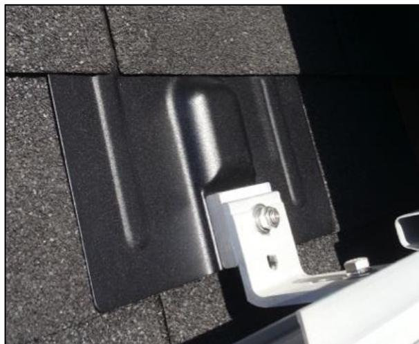
2. Prepare roof for installing lag bolts by drilling two 7/32" pilot holes through the roof and into the rafter for each base plate.
