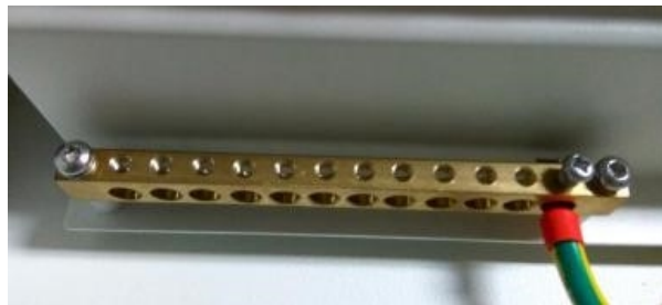
Figure 3.9 Grounding terminal block on the metal bracket
